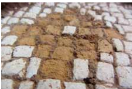
Figure 28 Detail of tesserae disaggregation.
