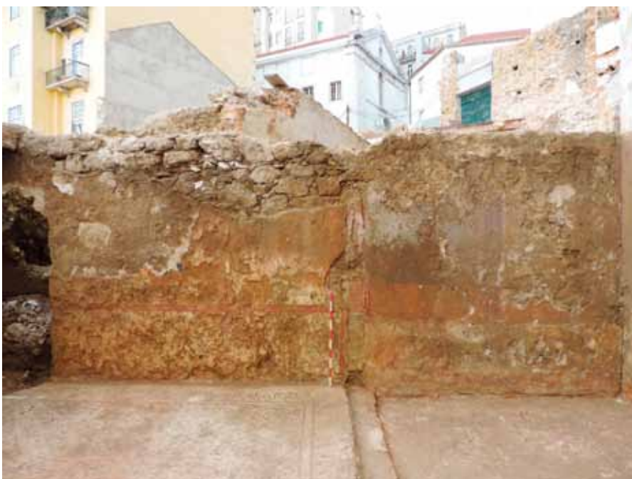
Figure 4 North wall painted plasters
