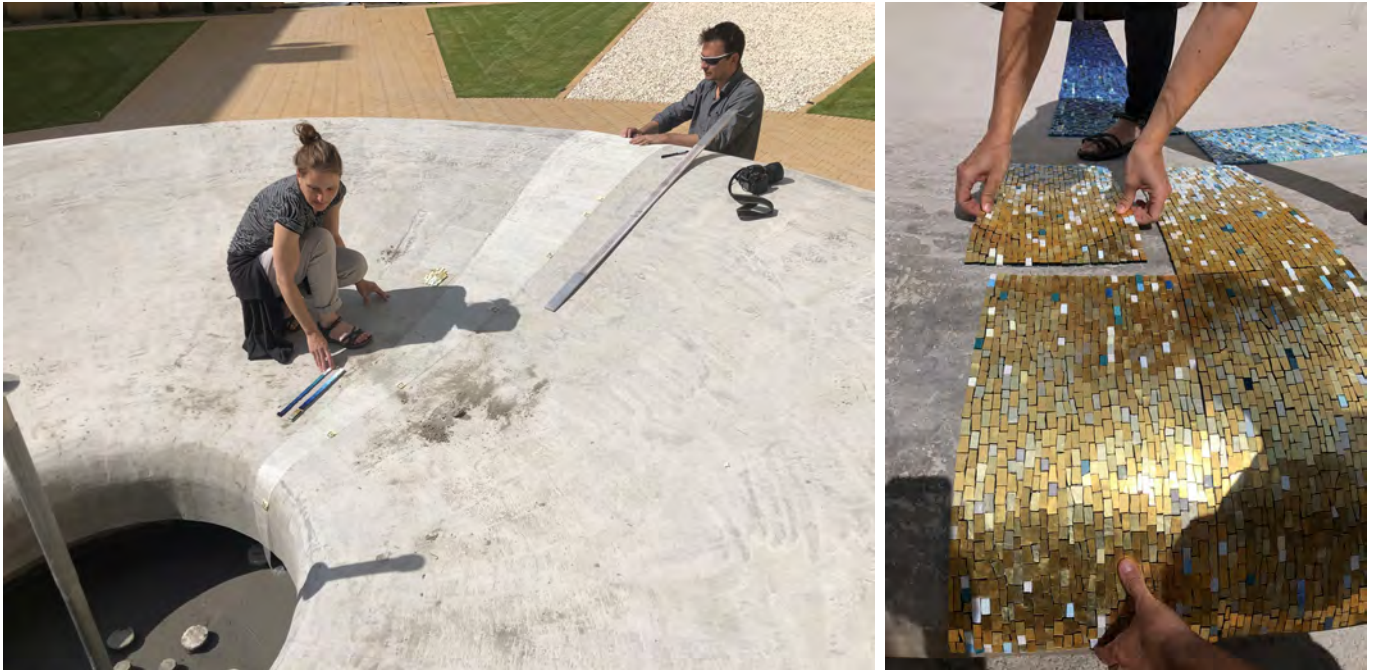
Figures 9a-b On-site measuring process for planning the best fitting size of the elements and trial to the arrangement of the firstly made sections following the measurements. Photos by Márta Vörös.
