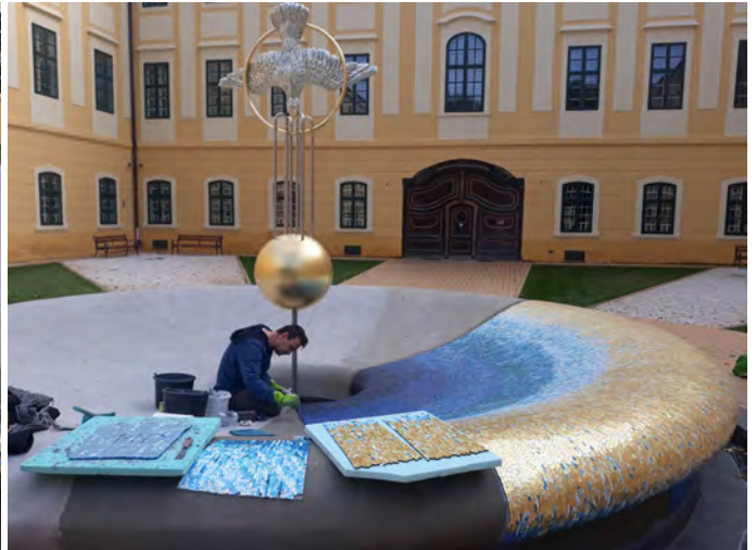
Figure 11 The embedding and the grouting process is made at the same time. The same material is applied on the backside of the mosaic section and on the surface of the fountain as well. Photo by Béla Dohárszky.
