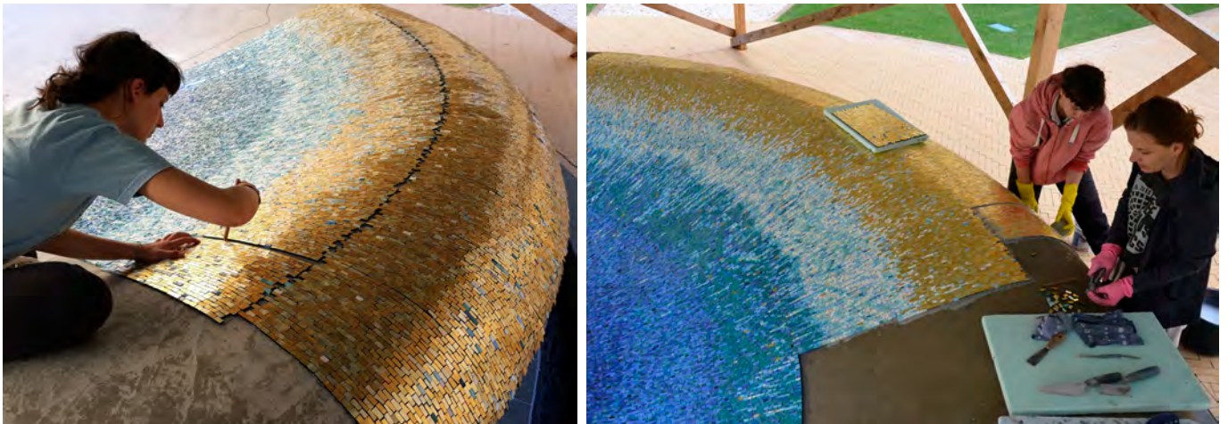
Figures 10a-b Drawing of the border of the sections for planning the extent and location of the on-site completions needed due to the slight irregularity of the fountain body shape. And the mounted and completed sections after the process. Photos by the author.
