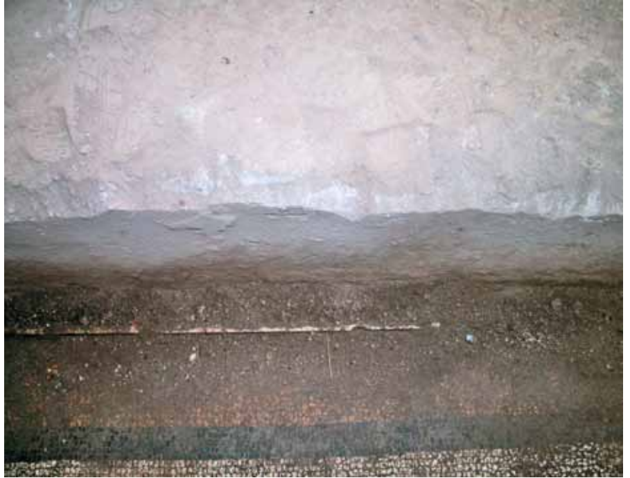
Figure 3 The tibuli system built in front of the wall
