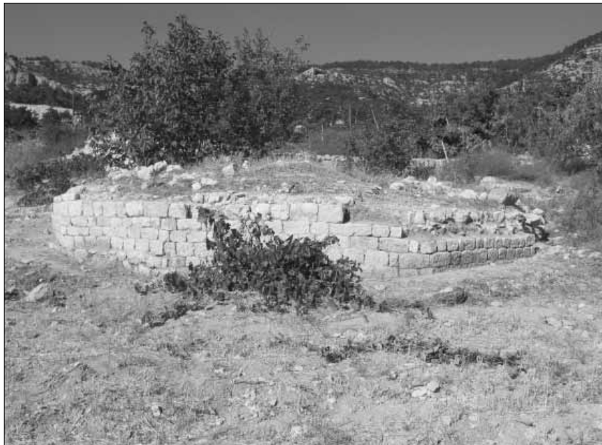
Fig. 6: Alahan tower (F373)
