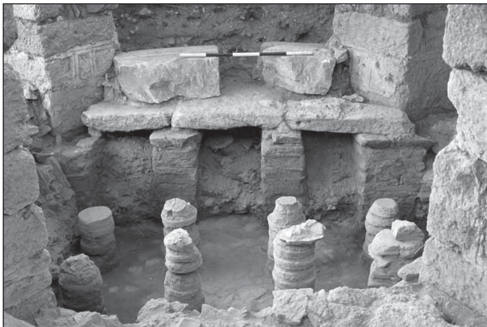
Fig. 11: The Tetraconch. View from the east of the western section of the hypocaust and suspensura of the central bay.
