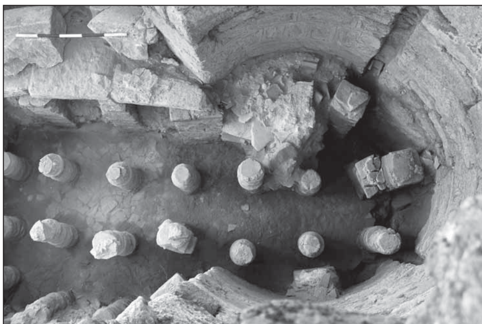
Fig. 12: The Tetraconch. View over the pilae and rock-cut channel in the northern apse .
