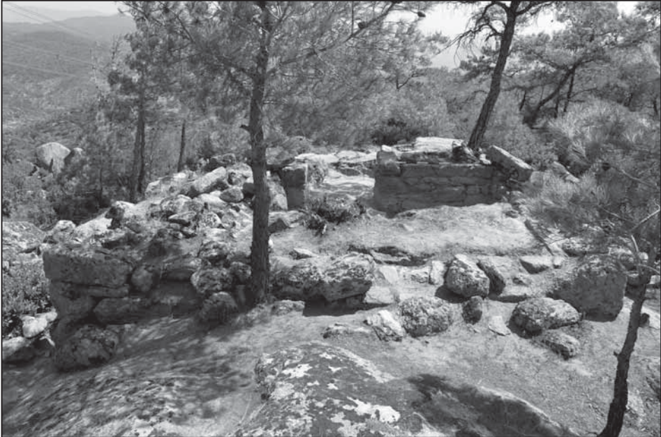
Fig. 8: View of the tower at Ucalan Kule from the north.
